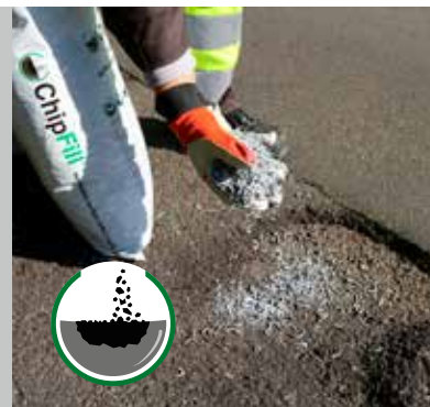
Apply a maximum initial ½ inch layer in the area.
