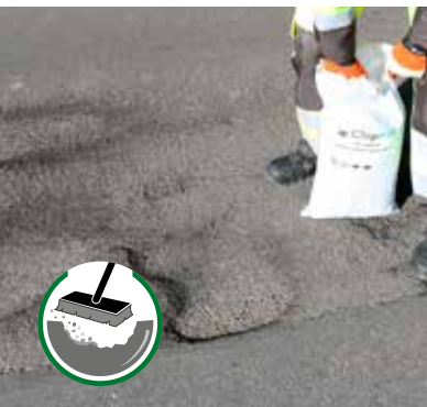
Remove debris and clean the repair area thoroughly.
