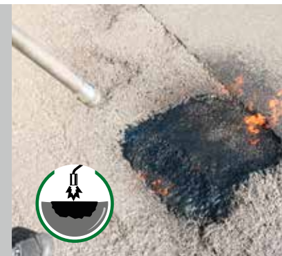
Heat material thoroughly and repeat process as necessary.
