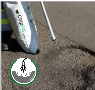
Remove moisture with a propane fueled heat gun.
